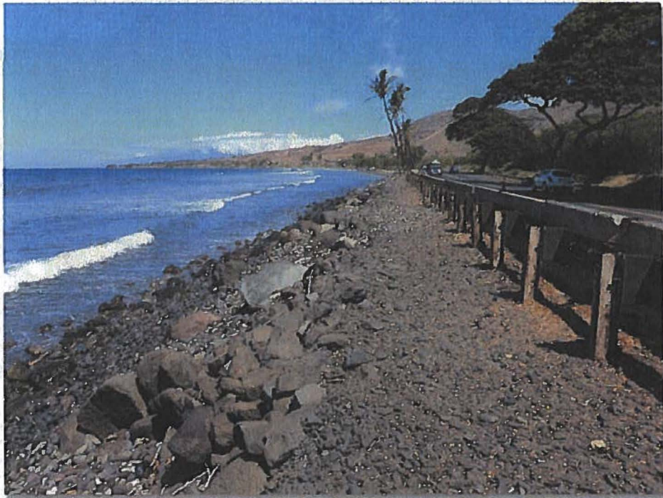
View of project site, looking west (toward Lahaina town). An emergency repair measure was constructed in 2009, shown in this photo taken in 2012.
