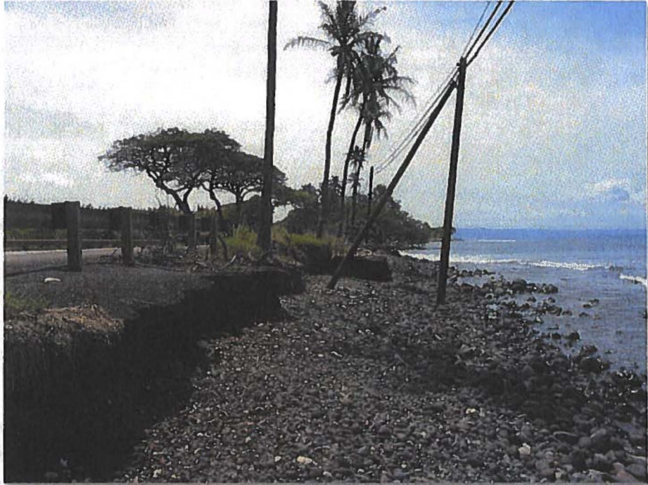
View of the project site, looking east. Photo taken in 2009.
