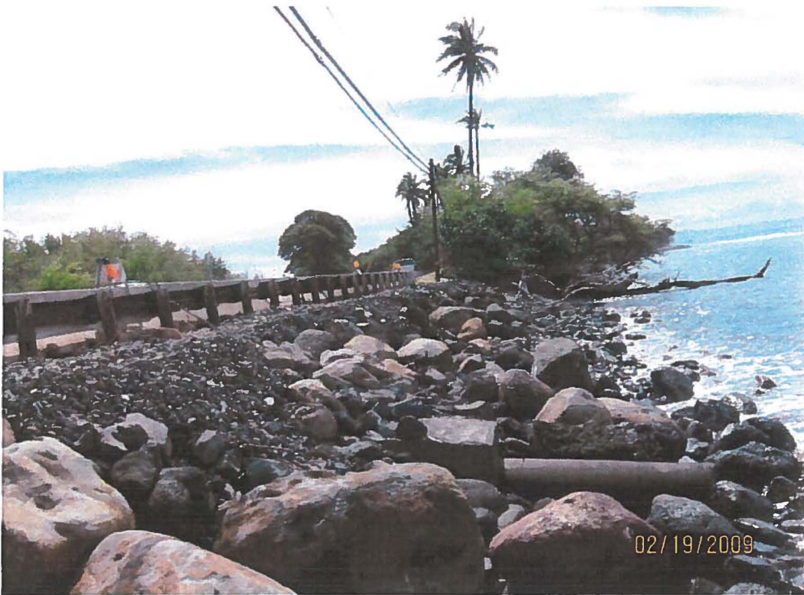
PHOTO NO. 1 - South View of Project Site; Honoapi`ilani Highway on left. Existing drainline in foreground
