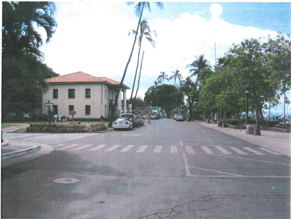
PHOTO NO. 1 - Wharf Street, South View
