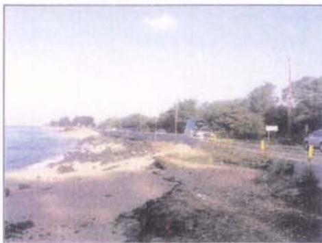
Protective barrier's located on the highway near Ukumehame Firing Range.
