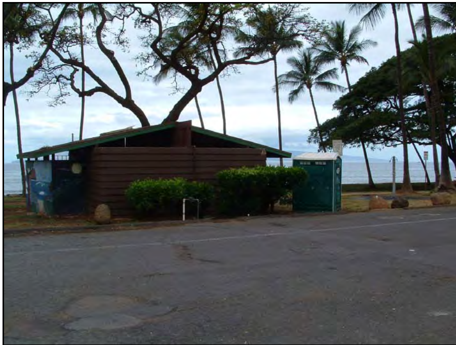
Figure 10. Launiupoko Beach Park, showing bathroom and shower facilities
