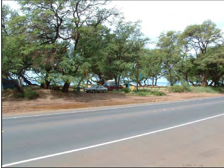
Figure 7. Pāpalaua Beach Park, showing graded area and railings
