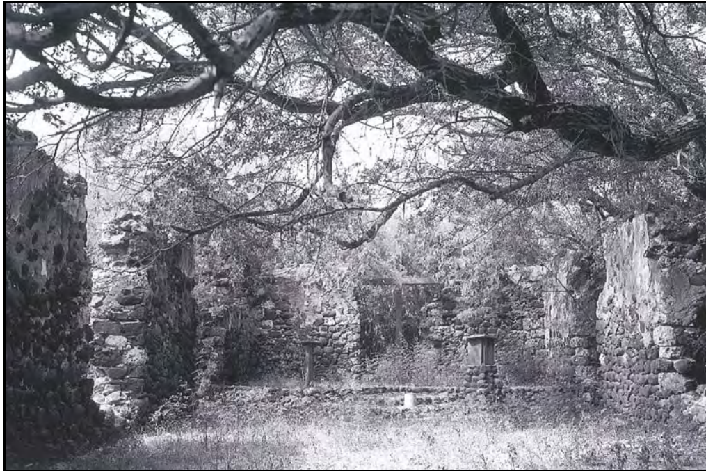
Figure 19. General Interior View of the Olowalu Church, photographed by Jack E. Boucher in 1966 for the Historic American Buildings Survey (HABS), and the Historic American Engineering Record (HAER) (National Park Service).
