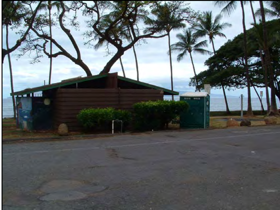
Figure 9. Launiupoko Beach Park, showing bathroom and shower facilities
