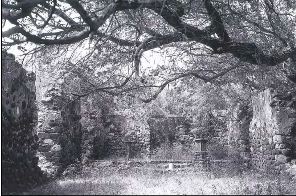
Figure 15. General Interior View of the Olowalu Church, photographed by Jack E. Boucher in 1966 for the Historic American Buildings Survey (HABS), and the Historic American Engineering Record (HAER) (National Park Service).
