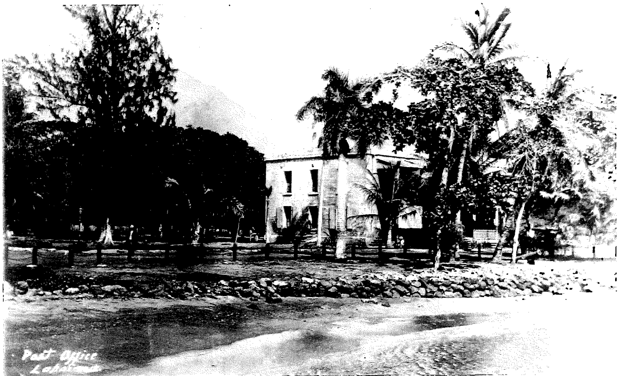
Figure 7 View to East Showing Low Retaining Wall and Large Trees on Courthouse Grounds
