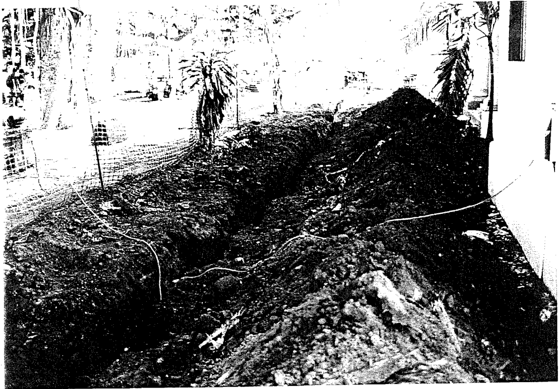
Trench for root barrier on east side of building—looking south.
