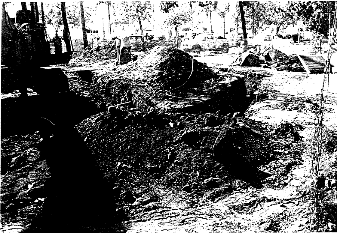
Subsurface excavation on north side of building.
