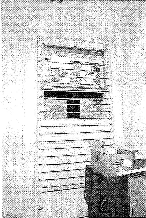
Figure 29. Bars on window in later holding cell
