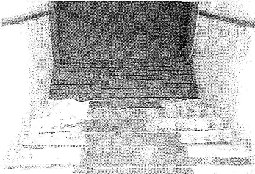
Figure 14. North stair to basement
