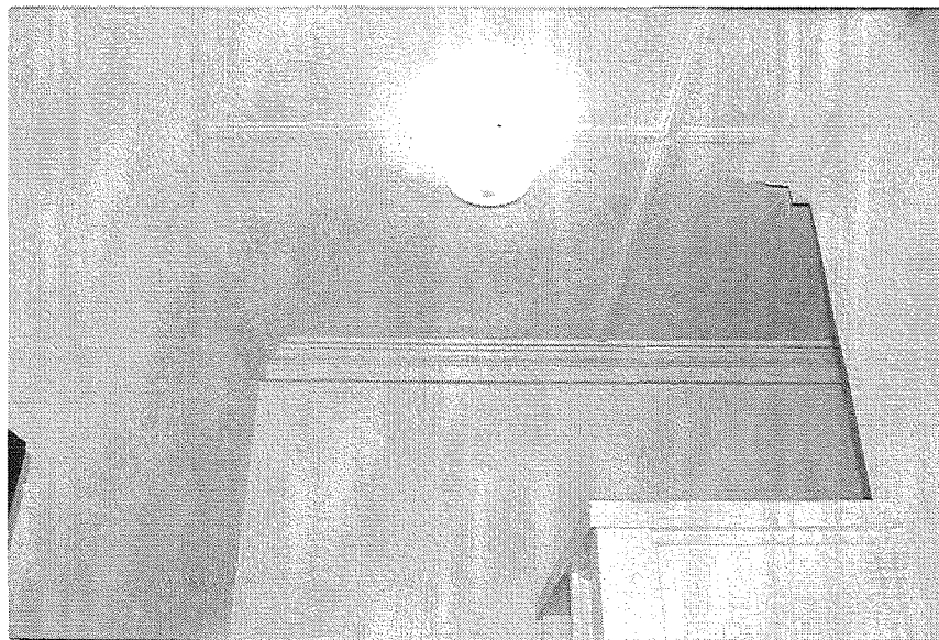
Figure 21. Ceiling in toilet room
