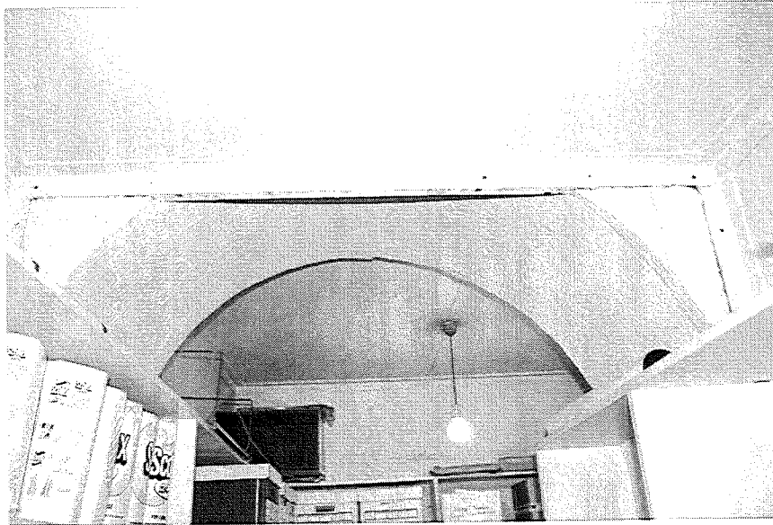
Figure 18. Opening to addition
