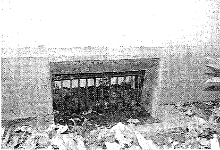
Figure 20. Vent opening to basement
