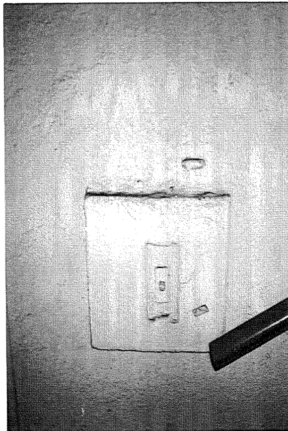
Figure 19. Latch strike at basement entrance
