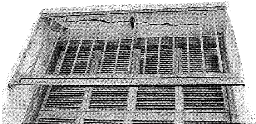
Figure 11. Crack at window lintel
