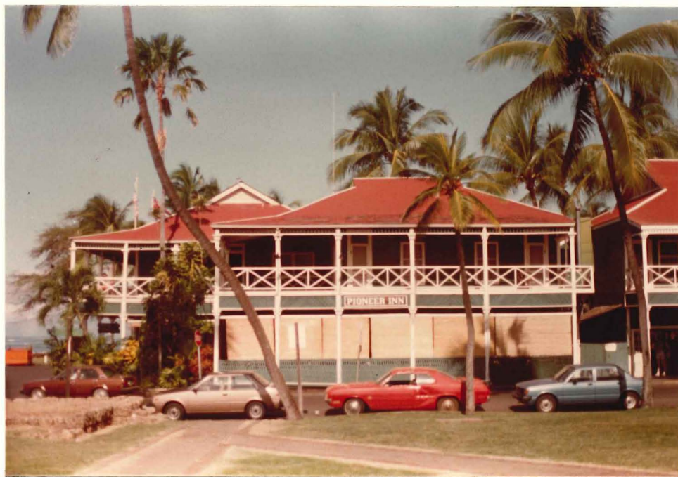
PHOTO OF ELEVATION - HOTEL ST. SIDE
